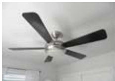
Installation of new ceiling fans
