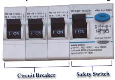
Typical switchboard – this shows the main switch, safety switch with test button and circuit breakers. All homes have circuit breakers or fuses. These are designed to protect the wiring and appliances within the premises. Only safety switches are designed to protect people.
