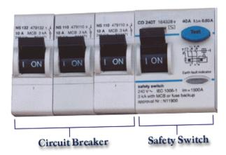
Typical switchboard – this shows the main switch, safety switch with test button and circuit breakers. All homes have circuit breakers or fuses. These are designed to protect the wiring and appliances within the premises. Only safety switches are designed to protect people.
