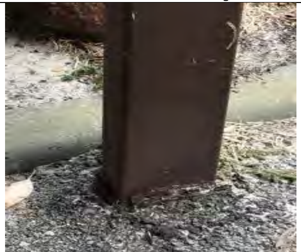
Close up view of steel post to Western corner showing advanced rusting below ground level
