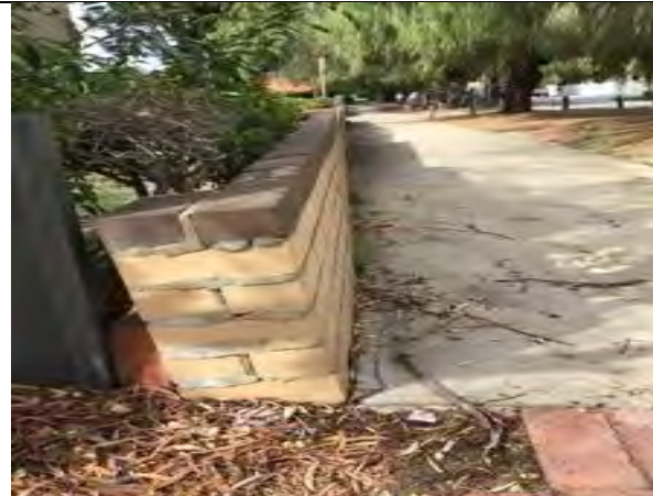
View of front boundary wall looking South Westwards, leaning evident
