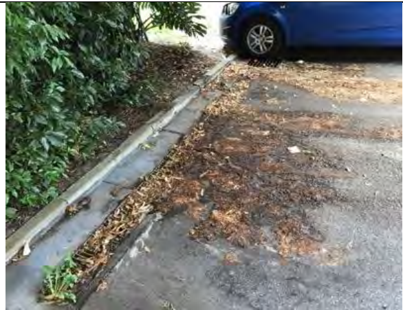
Trench grates blocked with soil
