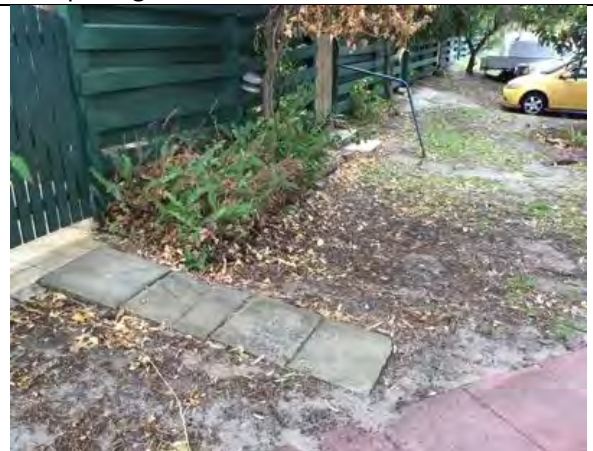
Substandard steps and pathways coming from Lots 1 to 8 courtyards down to parking level
