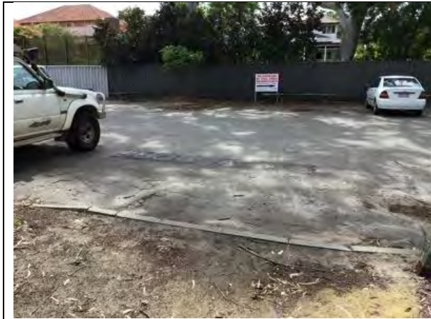
Bottom parking in the South East corner, bitumen in poor condition, drainage nonexistent and kerbs have collapsed
