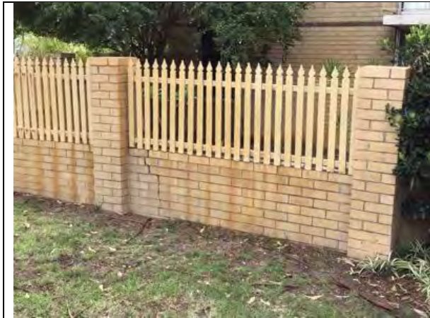
Cracking to South, Western corner of Lot 10 courtyard wall. Indicating settling of foundations to area. Requires underpinning & repair
