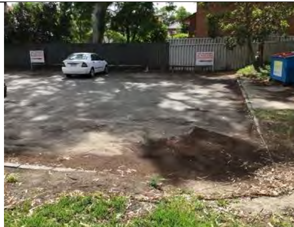
Soil build up collecting at base of Eastern carpark, no drainage visible
