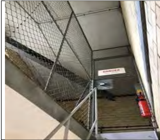
Top of steel staircase leading to lift plantroom, showing mesh fencing enclosure. Recommend lift installer provide new sealed, enclosure walls & access door
