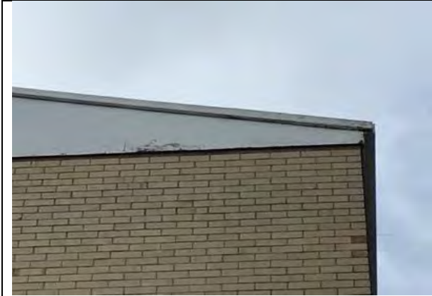
Close up of gable clad in ACM
