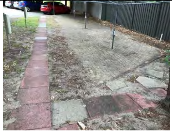
Continuation of pathway to lower parking and washing lines, substandard, remove and install new paving
