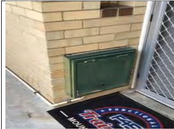
Pipe junction boxes outside each apartment, repair and repaint
