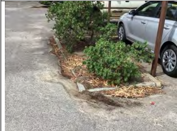
Collapsed Kerbs, damage and soil collection from run off
