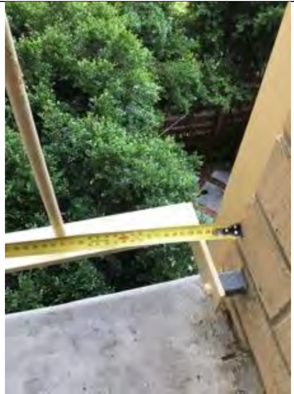
Gaps at walls in some locations are up to 200mm & non-compliant. Install extra balusters – Approx. 20 locations
