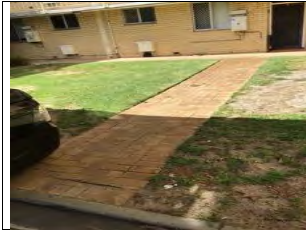
Pathway from upper parking, uneven in places
