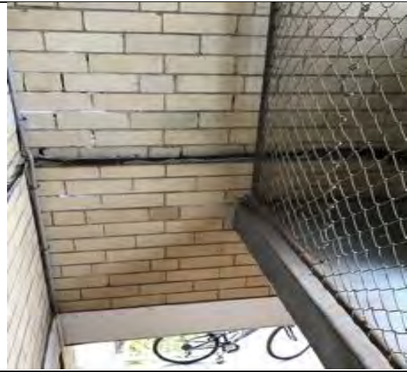
Rusted flashing junction, noted for replacement under exterior walls - brickwork
