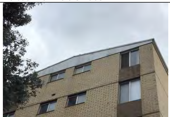
End elevation showing typical Gable end clad in ACM
