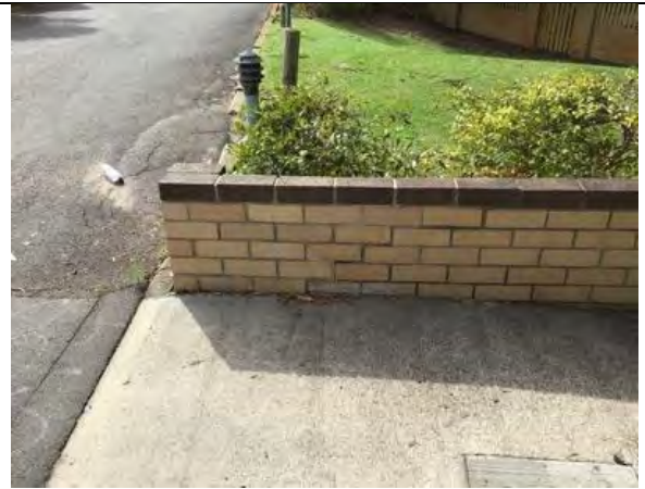
Evidence of vehicular damage, cracking to front boundary wall, repair/replace as required
