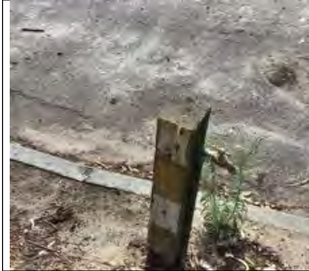
External taps fixed to timber post, vehicle damage risk. Recommend relocate onto carport posts
