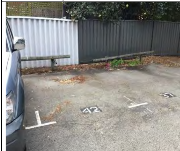
Eastern parking bays, faded line marking & timber vehicle stops are past their used by date
