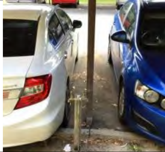
External taps fixed to timber post, vehicle damage risk. Recommend relocate onto carport posts
