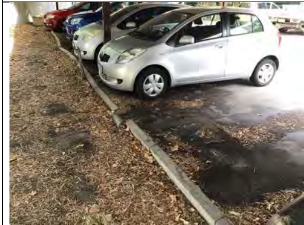
Collapsed kerbs and soil/debris build up running into drain
