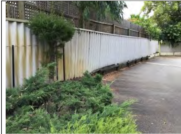
Further view of North Eastern section of fencing, section will require lower retaining panels included with the new fencing
