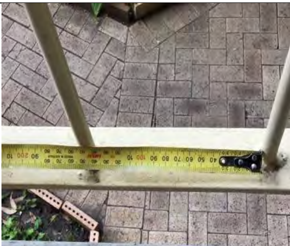
Common baluster spacings of approx. 150mm
