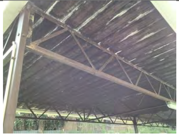
Carport structures are generally in poor condition, rusted framework structure and cladding
