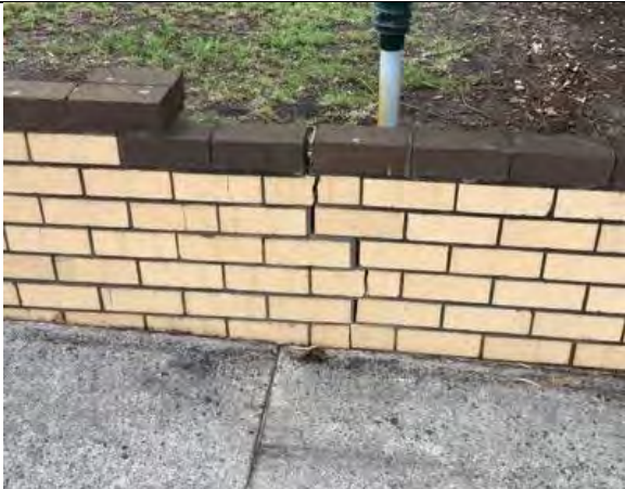
Evidence of cracking to Northern end of front boundary wall, repair/replace as required
