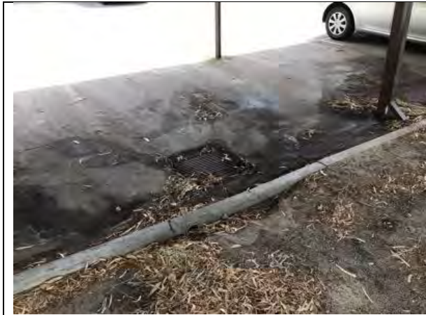
Soil run off built up against kerb & running into drain
