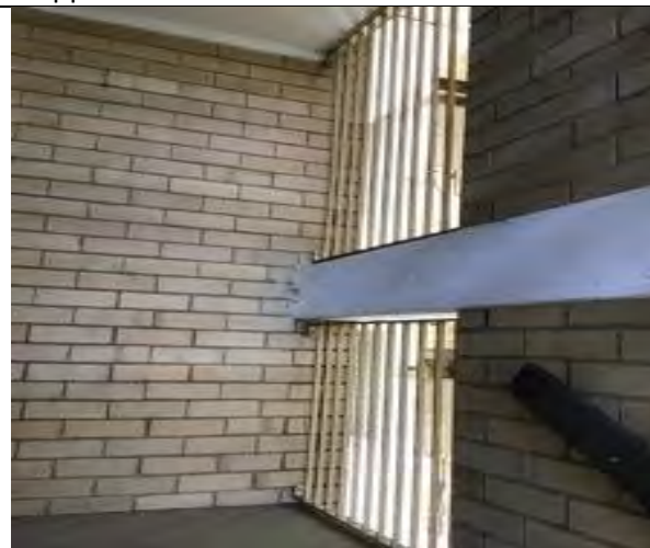
Balustrades at landings to Front stairs, surface rusting evident, prepare and paint
