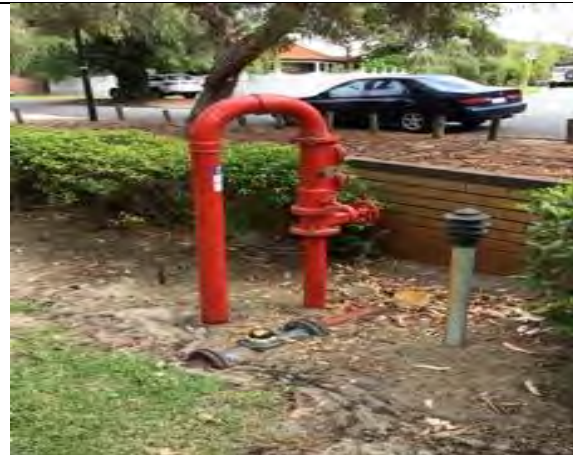
Fire main located in street side front garden
