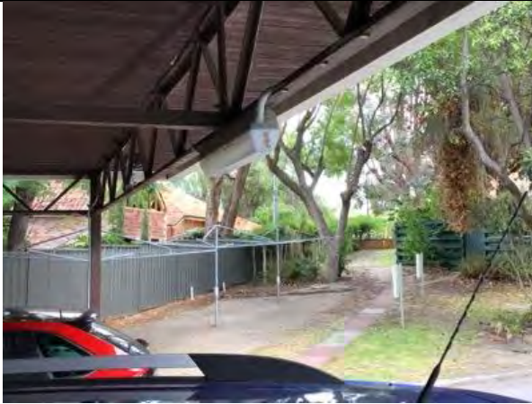
Fluorescent fittings to carports & floodlights to some parking areas
