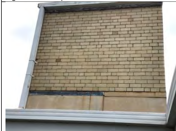
Rust deterioration to horizontal flashing to lift walls. Remove remaining material and replace
