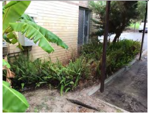
Ground build up against Northern end of Lot 10 external walls. Investigate potential moisture ingress internally
