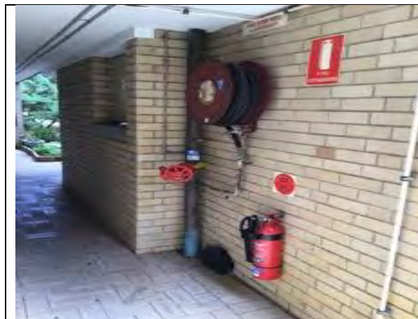
New Fire extinguishers located on each floor. Fire Hose Reels are rusted
