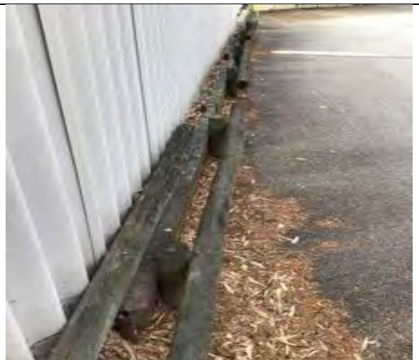
Deteriorated barrier to North Easter side, replace with steel barrier rail
