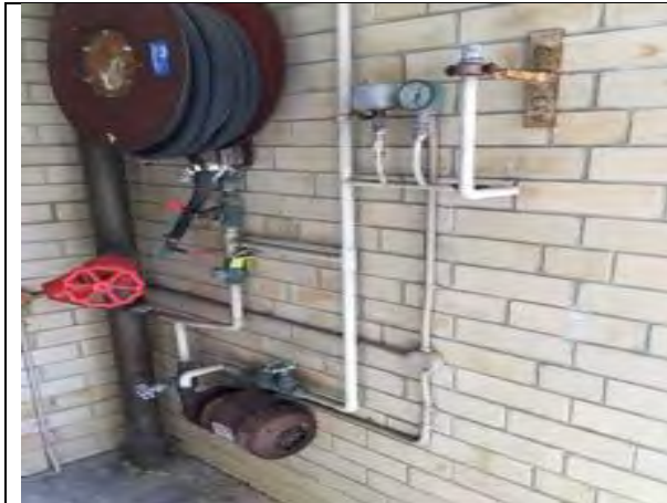
Pump below FHR appears to be in poor condition
