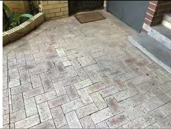
Low point in paving outside Lot 10 with unsatisfactory drain solution
