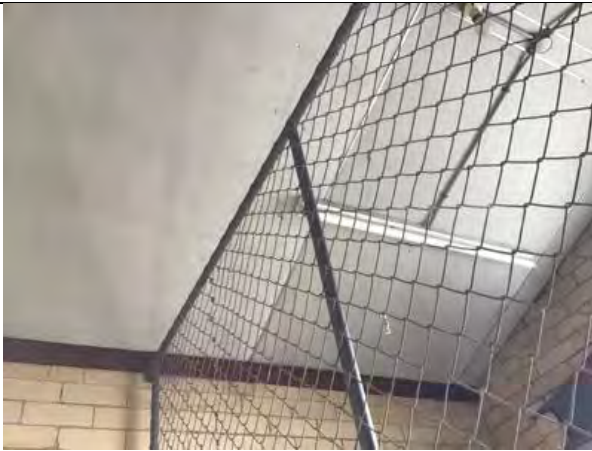
Asbestos ceilings, noted for replacement under eaves and ceilings
