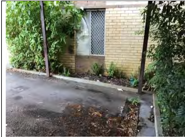
Ground build up against Northern end of Lot 9 external walls. Investigate potential moisture ingress internally
