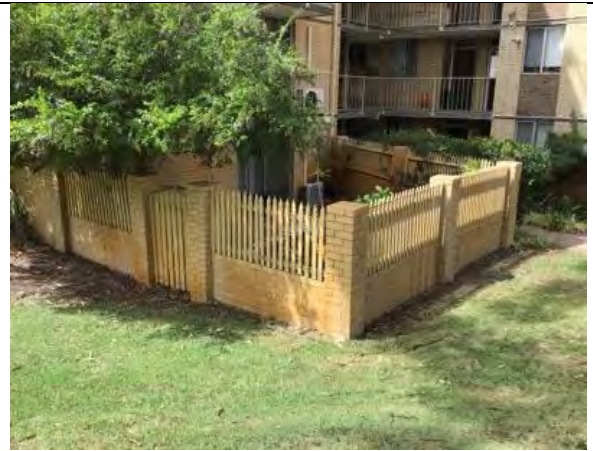
Courtyard to Lot 10 – Picket fencing requires remedial works and painting
