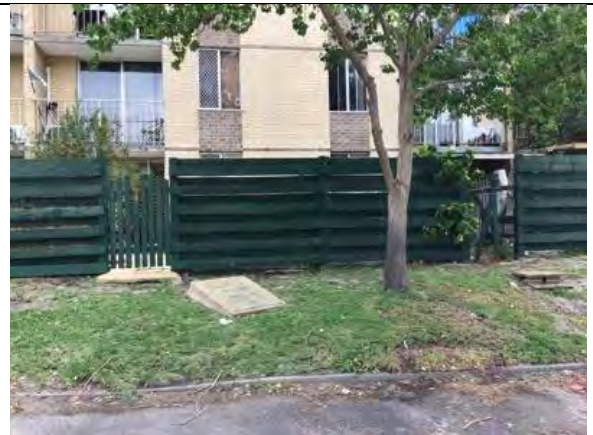
View of the front of the fencing showing missing/damaged access gates
