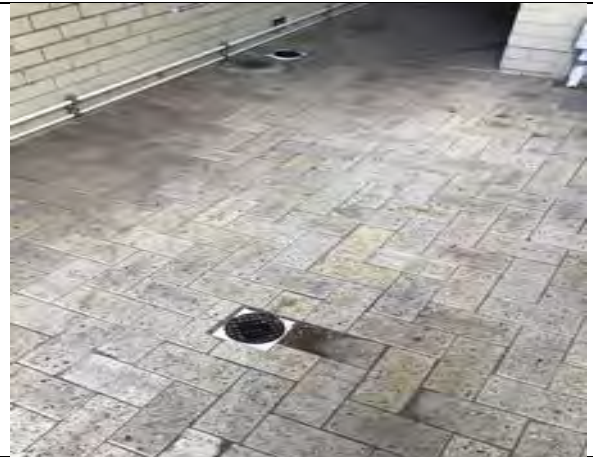
Paving to ground floor walkways, uneven in places & trip hazards around services
