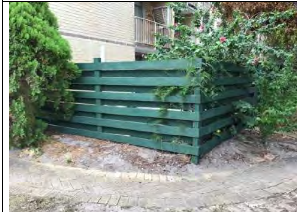
Timber fencing to Lots 1 to 9 has deteriorated, is rotten and collapsing. Requires replacing
