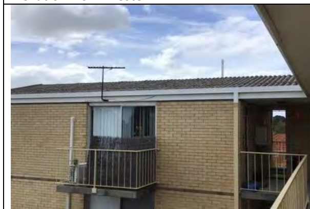
Roof over Lot 60 showing ACM roof cover
