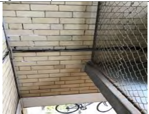
Internal view of deteriorated flashing to lift walls, remove and replace
