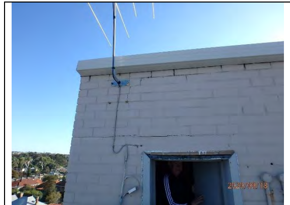
Access Door and Cracking to Lift Motor Room
