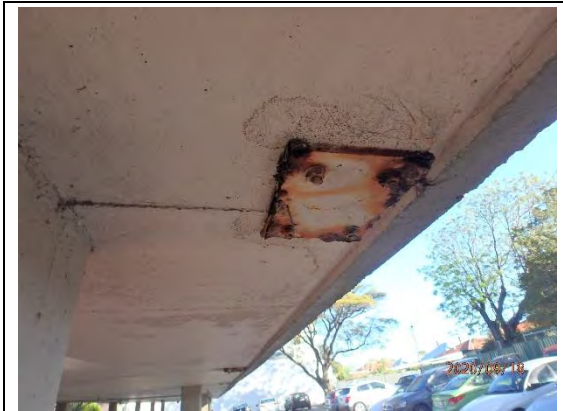
Corrosion to Base of Steel Columns
