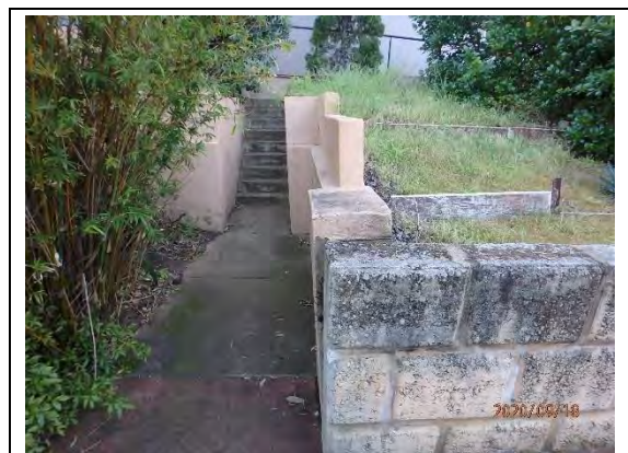
Retaining Wall Leaning
